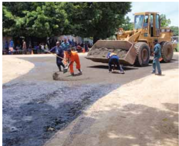
Grading and laying of bitumen for Daru Wharf road access.
