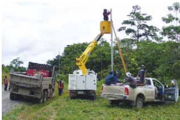
Erection of electricity poles for the Tutuwe Project, Rumginae, Western Province.
