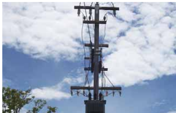
Step-up transformer at Rumginae Station connecting power to nearby villages, North Fly District, Western Province.
